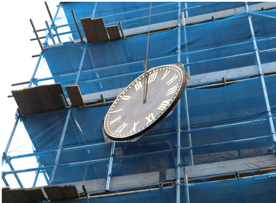
One of the clock faces from St Mary's being lowered for restoration. Photo credit : John Hunter
