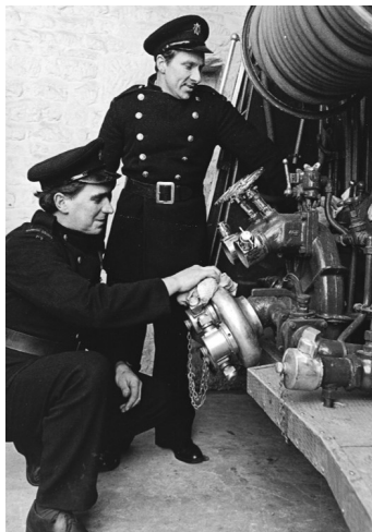
Firemen Pete Billing and Tony Lomas cleaning the pump inside the Fire Station, 1965.
